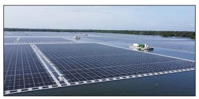
reservoir. Divided into 40 blocks, each having 2.5 MW. Each block consists of one floating platform and an array of 11,200 solar modules.
